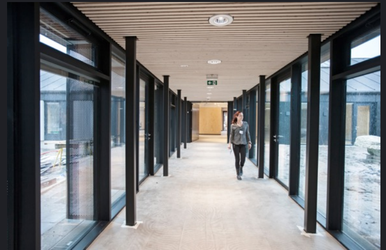
Connecting glass corridor
