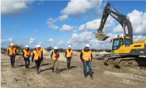
VINGE CONSTRUCTION SITE
